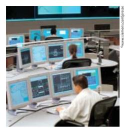
The Trainguard MT Communications-Based Train Control (CBTC) rail automation technology installed on the New York Metro enables trains to run at intervals of 85 seconds.
