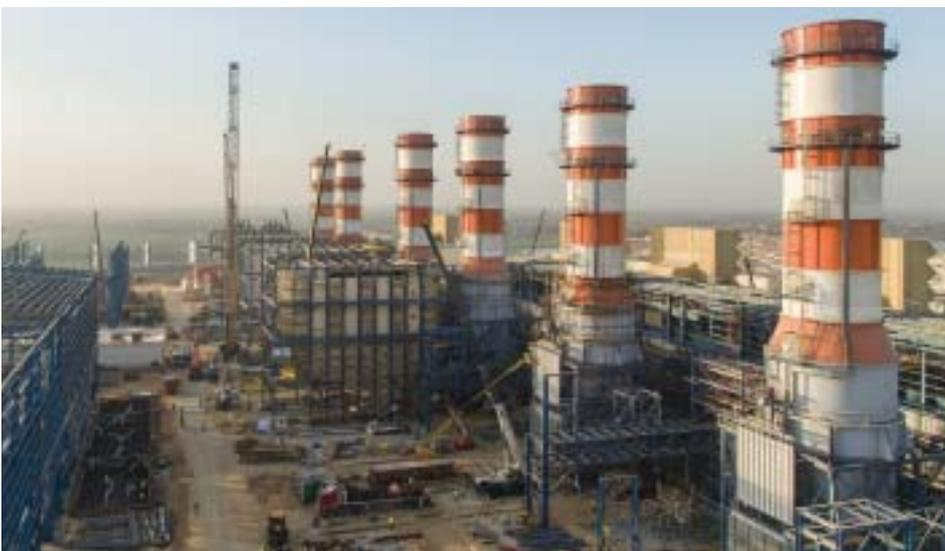
Together with its local Egyptian partners, Siemens is erecting three turnkey gas-fired combined cycle power plants, each with a capacity of 4.8 gigawatts, for a total combined capacity of 14.4 gigawatts.
